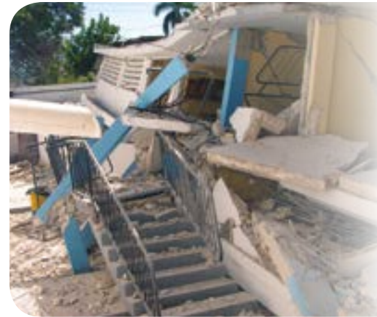
Devastation following the earthquake in Haiti
